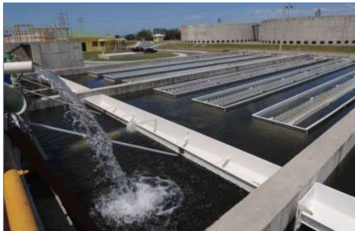
Manfouha Sewage Treatment Plant Project - Phase 4
